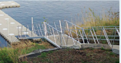
HANDRAIL INCREASES THE GANGWAY'S RIGIDITY AND SAFETY.
